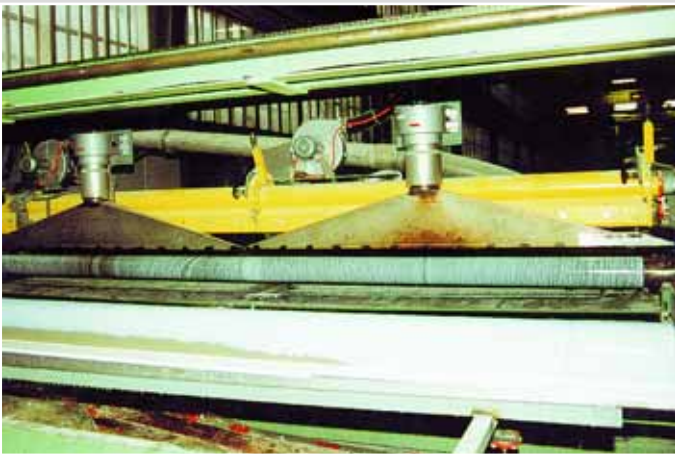
Two Heaters and two blowers used to dry impregnated Eternit piping. Two wide slot nozzles ensure the air is evenly distributed.
